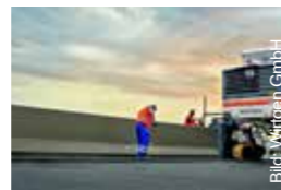
CONCRETE PROTECTION WALLS
